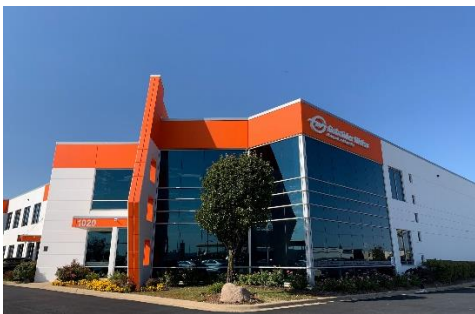
Caption: More space for employees and goods: the new US Head Office of Gebrüder Weiss in Chicago. (Source: Gebrüder Weiss)
