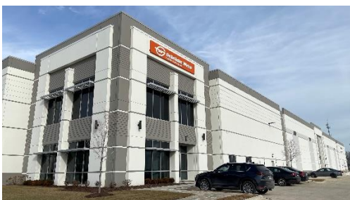
Caption: The new Gebrüder Weiss logistics warehouse in Chicago. (Source: Gebrüder Weiss)
