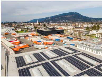
Caption: By 2030, Gebrüder Weiss plans to reach CO 2 neutrality at all its sites. Pictured here: the photovoltaic system at the Lauterach location, with Gebrüder Weiss headquarters in the background. (Source: Gebrüder Weiss / Sams)
